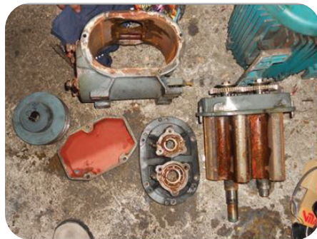
Overhaul the Root Blower
