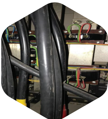
Lay power cable
