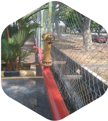
Lay & Install Hydrant Pipe System
