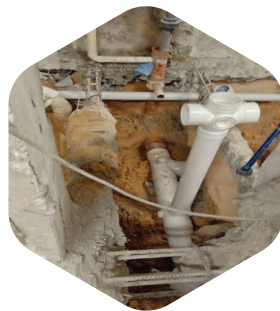
Lay underground Sewage Piping System
