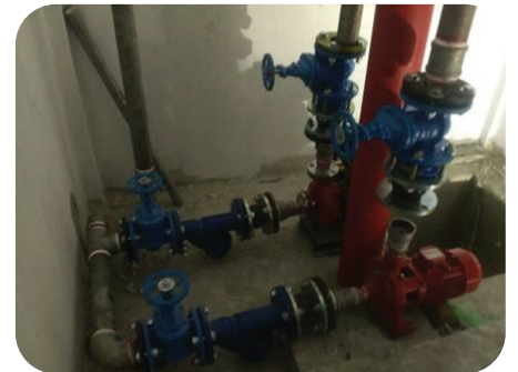
Installation of new pumps & valve on-site
