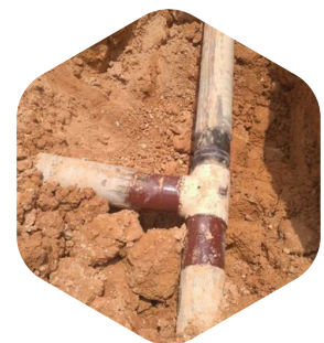
Lay Underground Domestic Water Pipe Line
