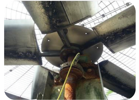
On-site servicing for Cooling Tower
