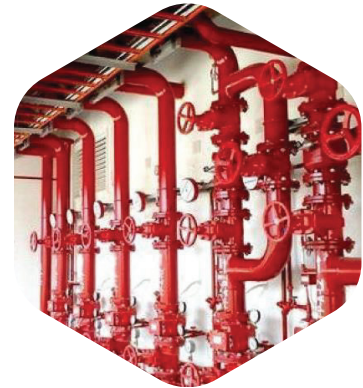
Lay Main Fire Pipe Line System
