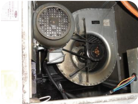
Servicing & repairing the FCU & AHU System
