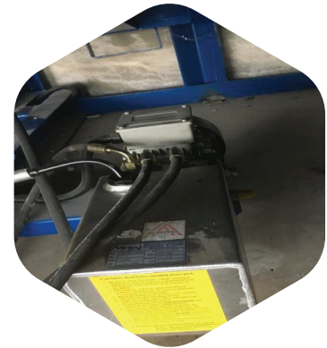
Supply & Install New Hydraulic Pump & System
