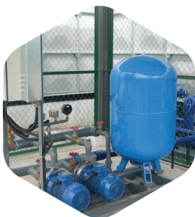
Installation of Domestic Water System
