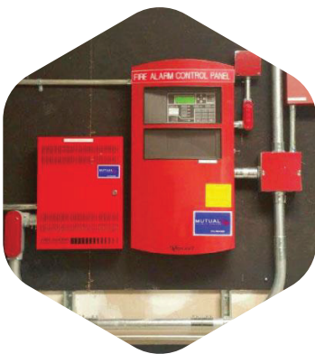
Supply & Install Fire Control Panel
