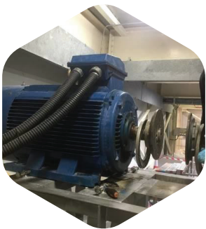
Installation of Heavy Rotating Mechanical Equipments
