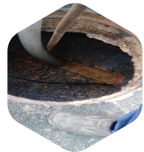
Grease Trap Installation
