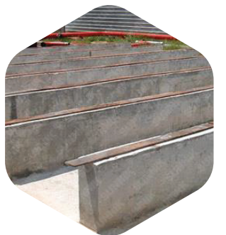
RC Plinth For Fire Tank
