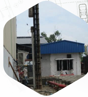
Piling & Structural Works
