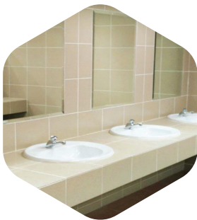
Upgrade toilet Sanitary System
