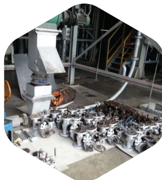
Boiler Valve & Part Overhaul
