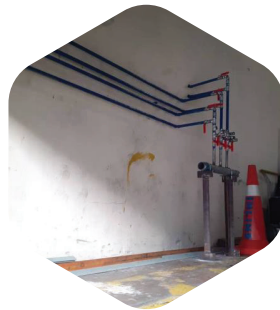
Lay New Compressor Air Piping
