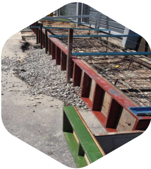
Concrete Construction Works
