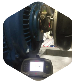
Perform Laser Alignment for Rotating Equipments
