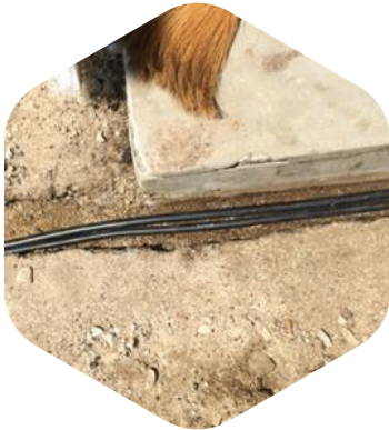
Lay underground power cable
