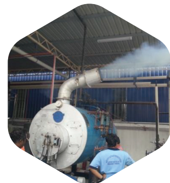
Boiler Test & Commissioning
