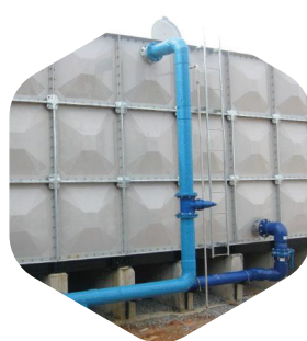
Supply & Install Domestic Water Tank & Pipe Line
