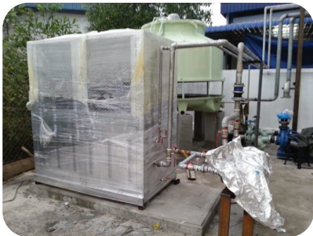
Installation of new Cooling Tower
