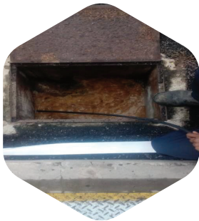
Hi- Pressure Jetting to clear pipe blockage
