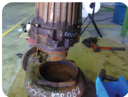
Repair & service all kinds of pumps
