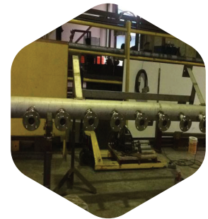
Boiler Steam Pipe Header Preparation at Yard
