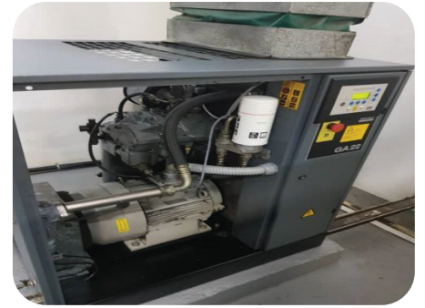
Overhaul Air Compressor
